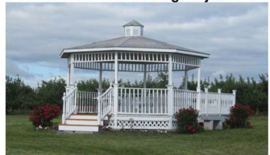
Gazebo Refurbishing Project
